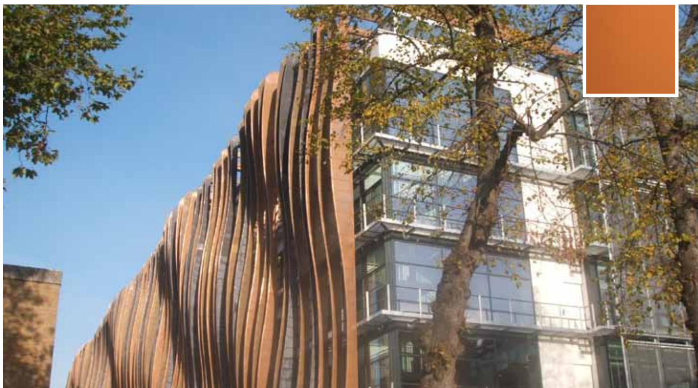
Vertical solar shading fins, each clad in either Nordic Bronze, Nordic Brass or Nordic Brown™. Holland Park School, London; Architects: Aedas.
