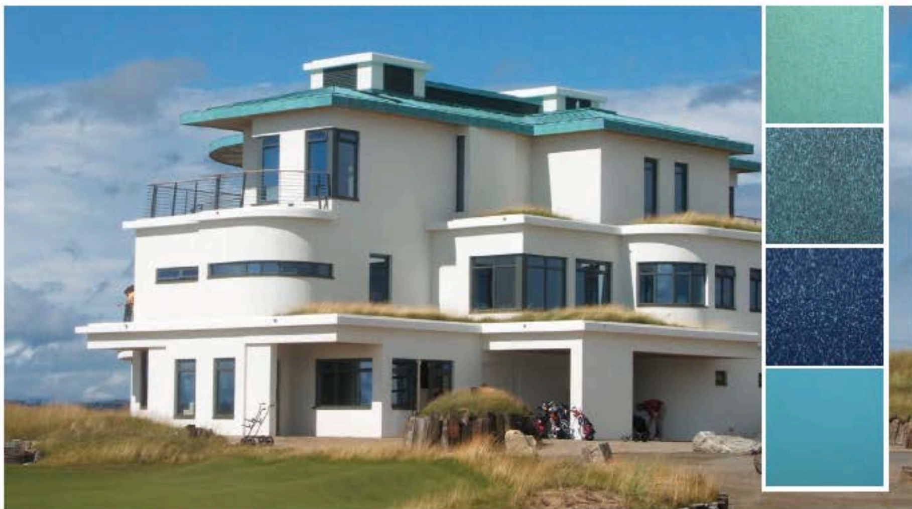
Castle Stuart Golf Links Clubhouse, Scotland; Architects: G+A Architects.
