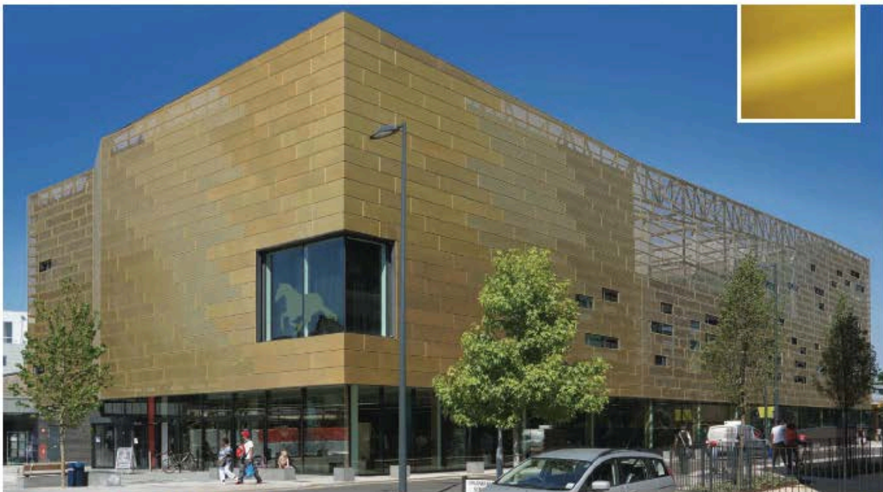
Deptford Lounge, London; Architects: Pollard Thomas Edwards architects.
